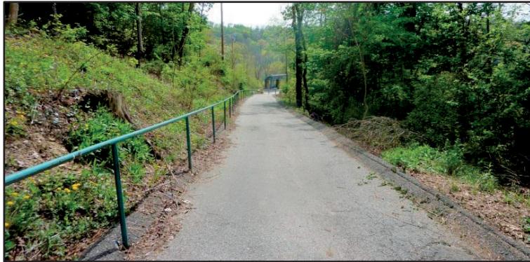
Figure 5: Walkway to Boggs Station
