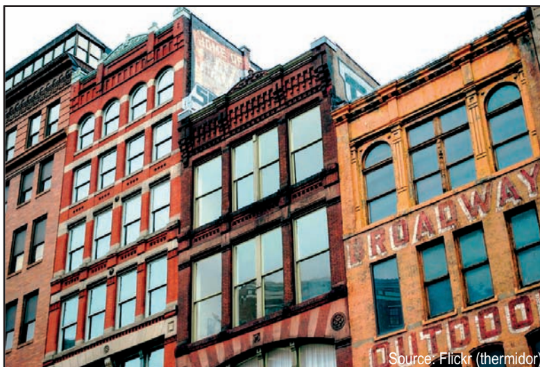
Figure 3: Historic building stock in downtown Pittsburgh
